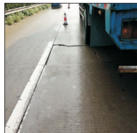
(c) 角隅断裂及错台板
