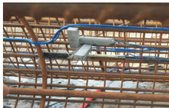
(a) 砼应变计安装于钢筋笼
