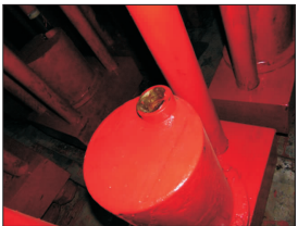
(b) 锚头防护帽油杯缺失
