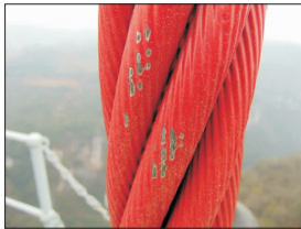
(a) 吊索涂层局部剥落
